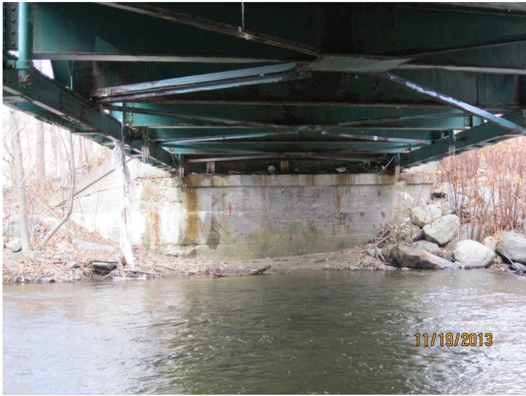
Picture 8: Northern Abutment
