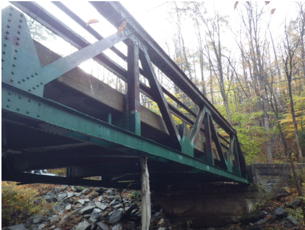
Picture 10: Upstream Bridge Fascia
