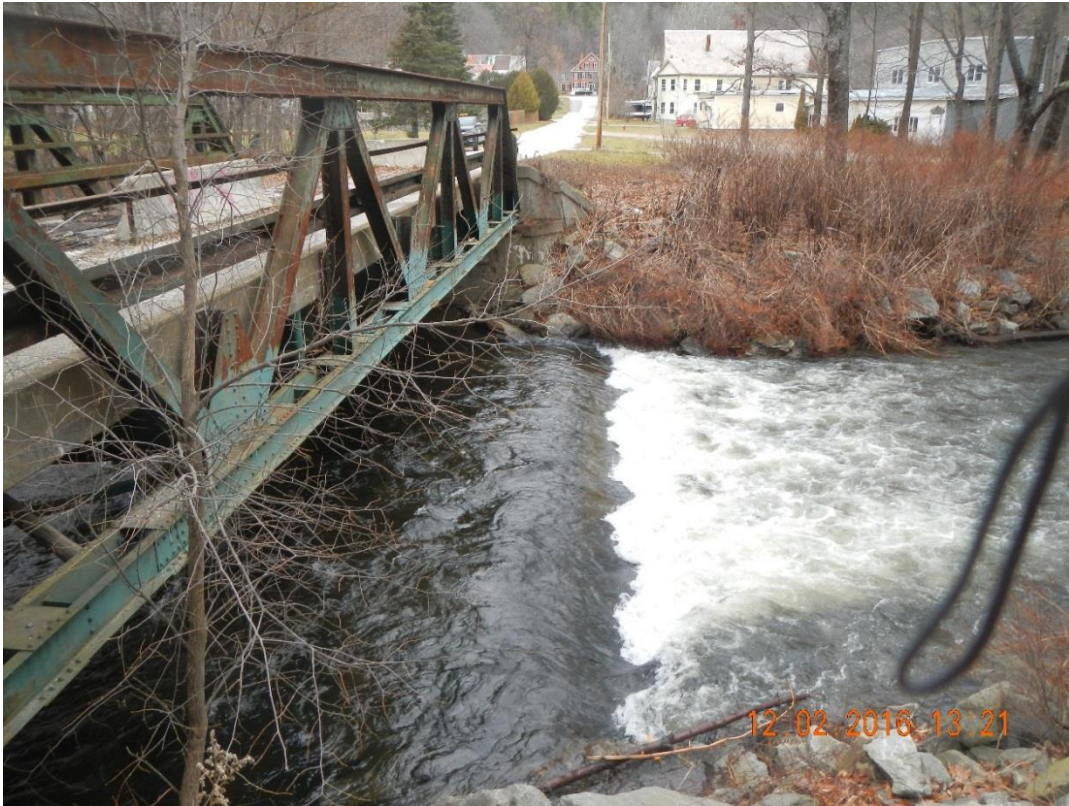
Figure 3: Cobbles and boulders within river and on river banks on downstream side. Also visible is possible weir within river.
