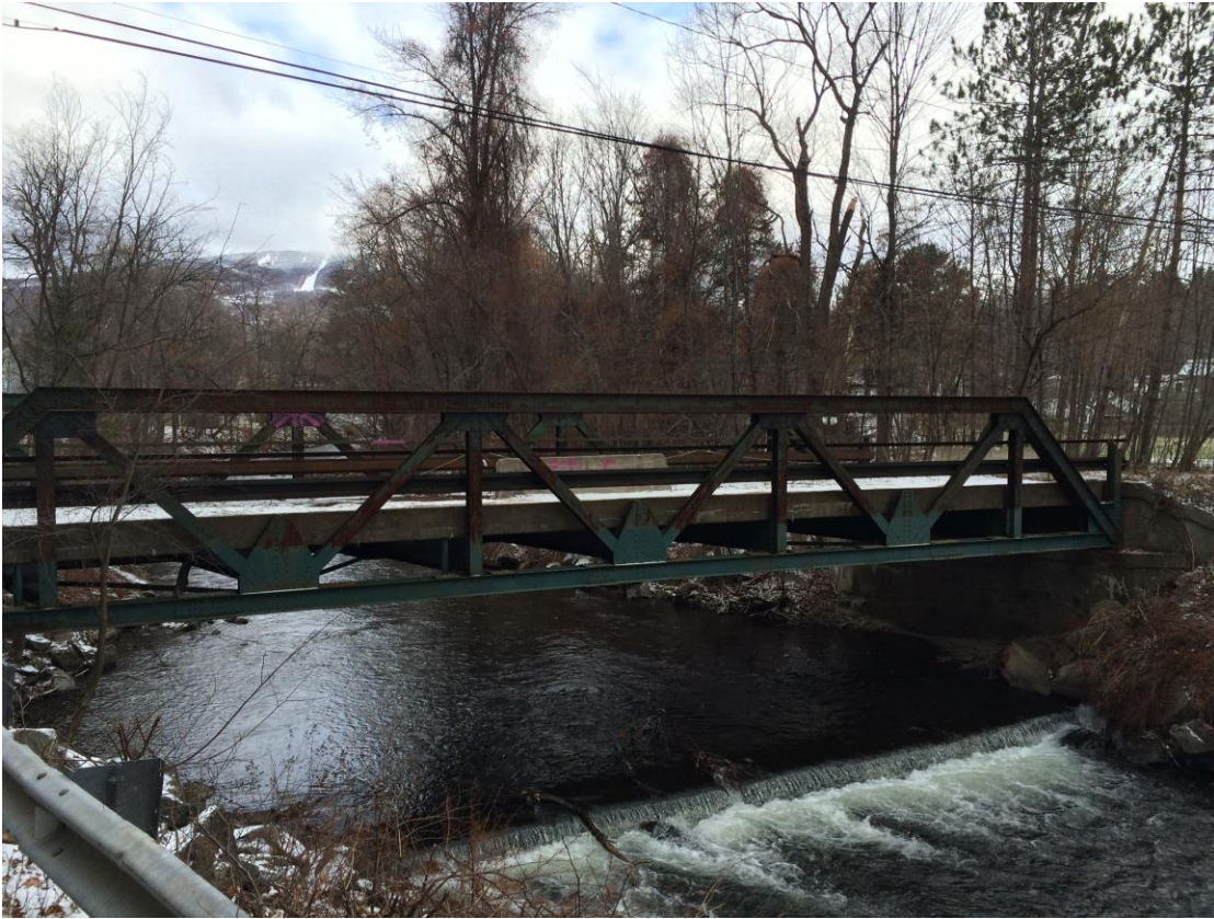
Figure 1: Bridge 57 View West
