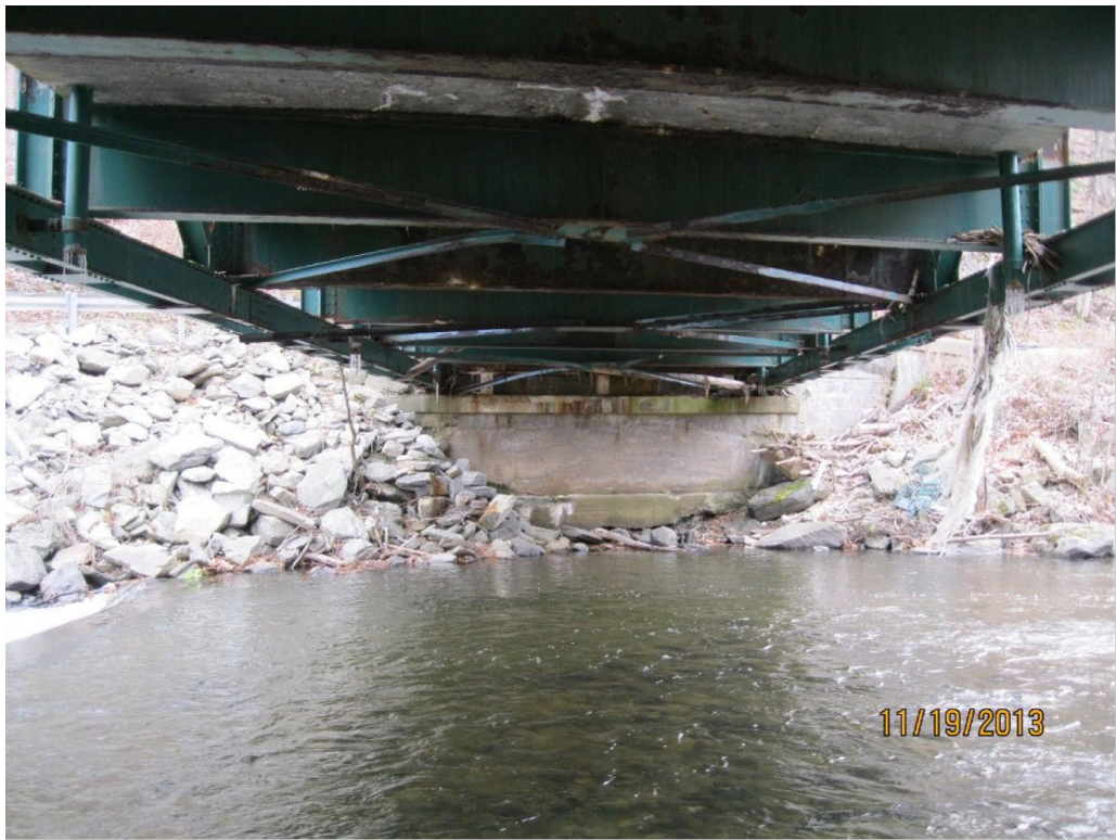
Picture 7: Southern Abutment
