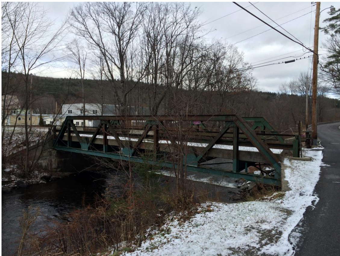
Figure 3. Bridge No. 57, looking east at the Black River from Pleasant Street.
