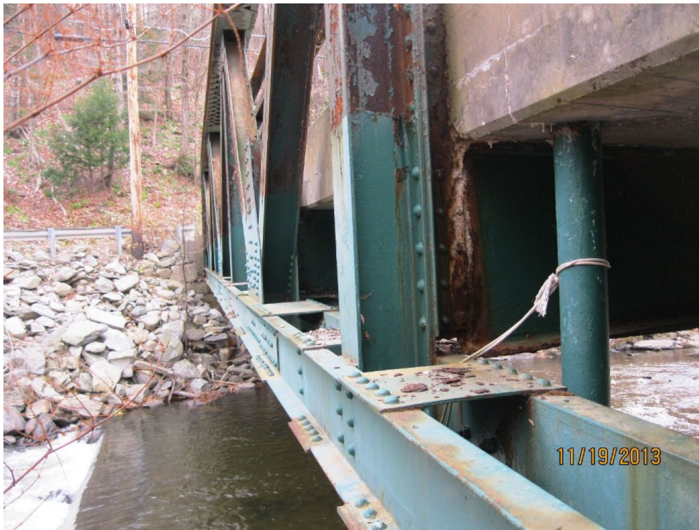
Picture 9: Downstream Bridge Fascia
