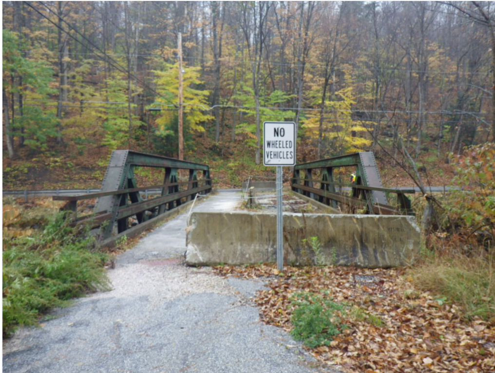
Picture 1: Looking South over Bridge 57
